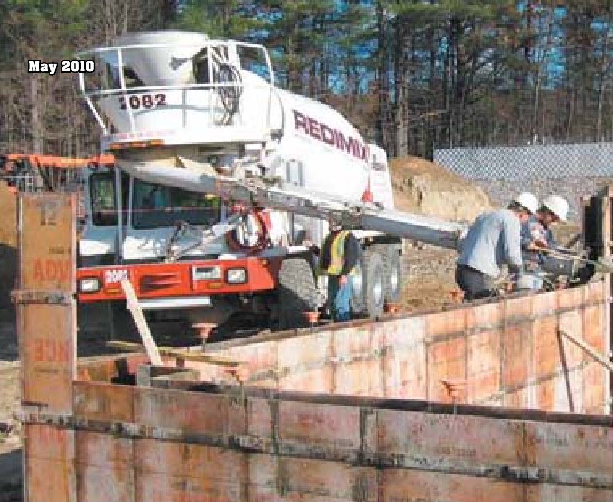
Tru-Form Foundation Inc. workers direct discharge of concrete from Redimix Companies' Oshkosh transit mixer for foundation wall.
