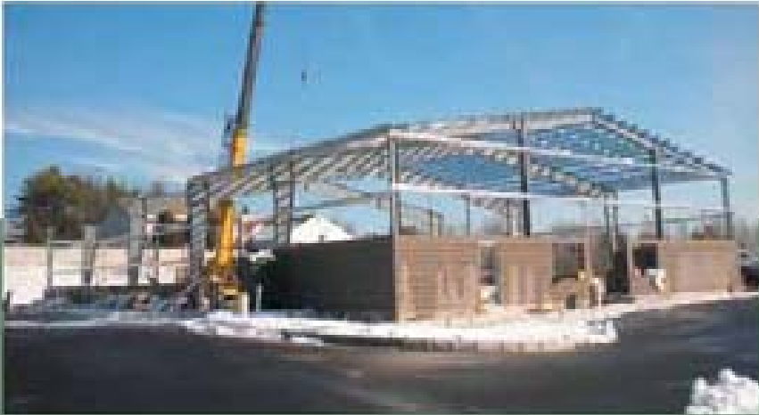
Building skeleton is nearly complete. Standing seam metal roof and siding will be placed next. Bigger photo: Erection crew attaches Butler's Shadowwall metal siding to horizontal girts.
