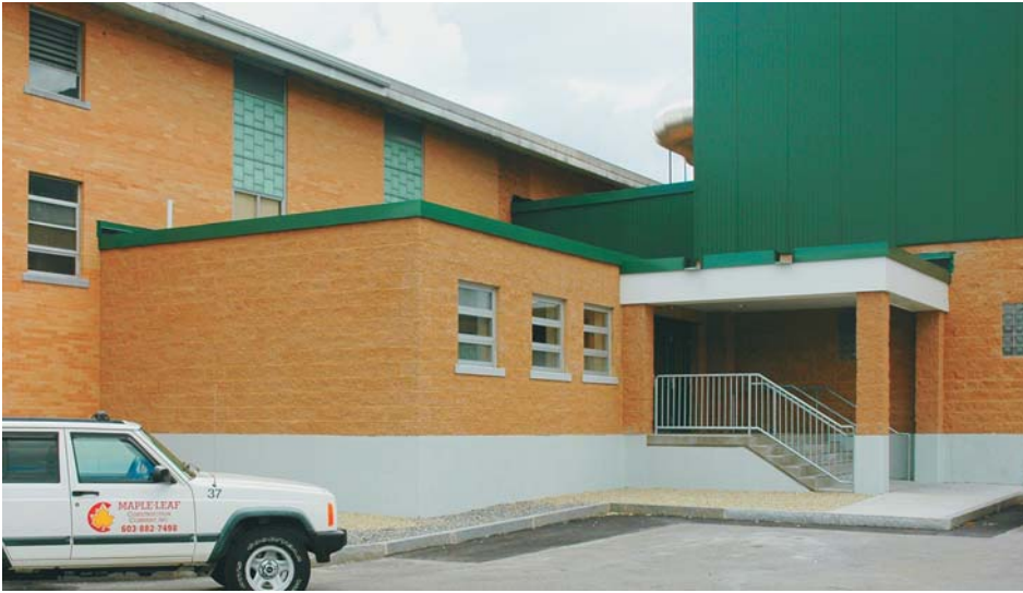
The field house restrooms at Bishop Guertin High School under construction.
