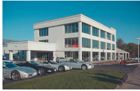
An alternate view of completed Phase II. New vehicles are shown on all three floors, as well as vehicle service canopy and exterior patio.
