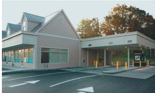
A look at the newly constructed drive-thru teller lanes. The entire drive-up area was constructed as part of the bank build-out package and designed with customer safety and security in mind, as well to blend seamlessly with the existing plaza's finishes.
